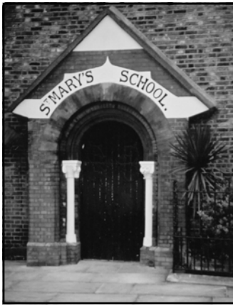
Entrance to the old school
